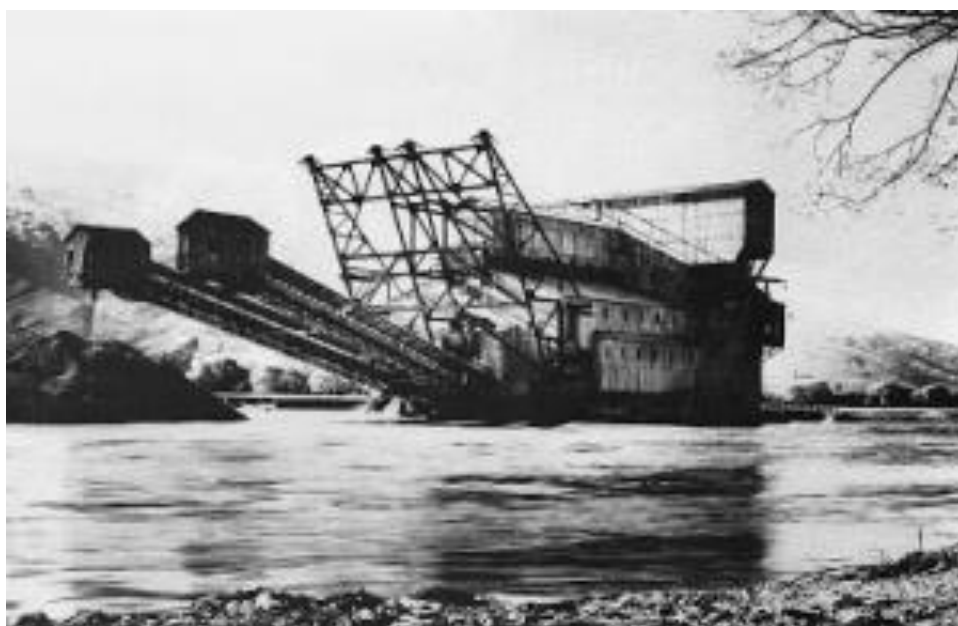
Austral-New Zealand’s massive dredge at Lowburn
