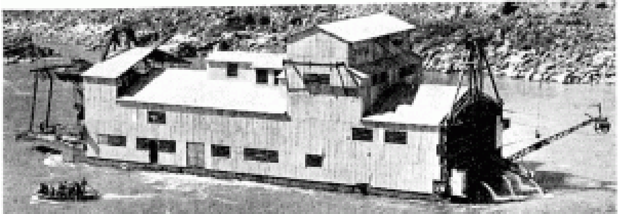
"Alexandra" at work on the Clutha River late 1930s, before extensions.
